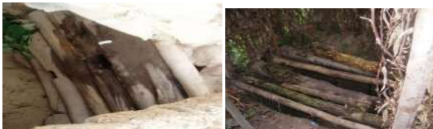
Figure 4 Some of the Pit latrines in Gahunga sector Burera district
