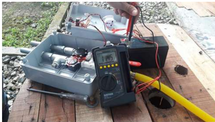
Fig. 10:- Battery voltage after charging 15 minutes without using current booster.
