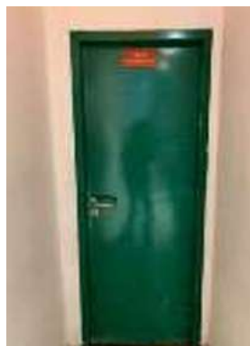
Figure 13:- Life Safety Facility - Emergency Doors at Lampung City Mall.
