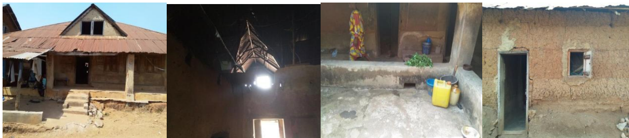
Figure 3.a, b, c, d:- Raised Entrance with dormer roofThe impluvium Courtyard and back earthen wall and openings.
