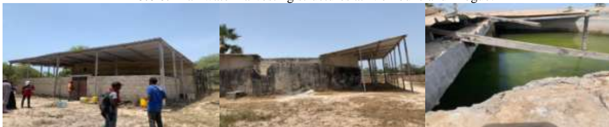
Photo 6:- Rainwater harvesting structures at Niomoune and Diogu .
