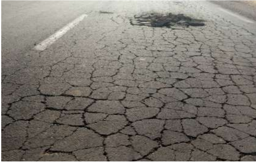
Figure 3:- Pavement crazing.
