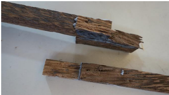
a) Cohesive breaking in the substrates
