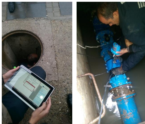
Fig.2:- a)Setting up the device. Fig. 2:- b) installing into main pipes.
