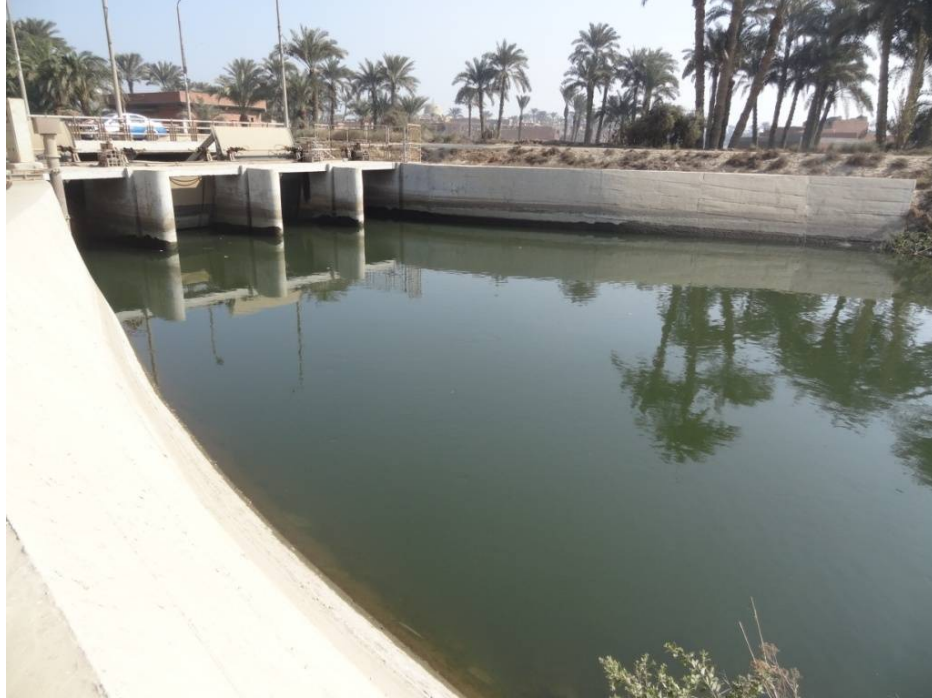
Photo5:- U.S. View of ST-5 shows fully closed two gates and fully opened two gates
