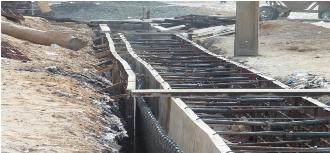
Figure 3:- Completed segment ready to be casted
