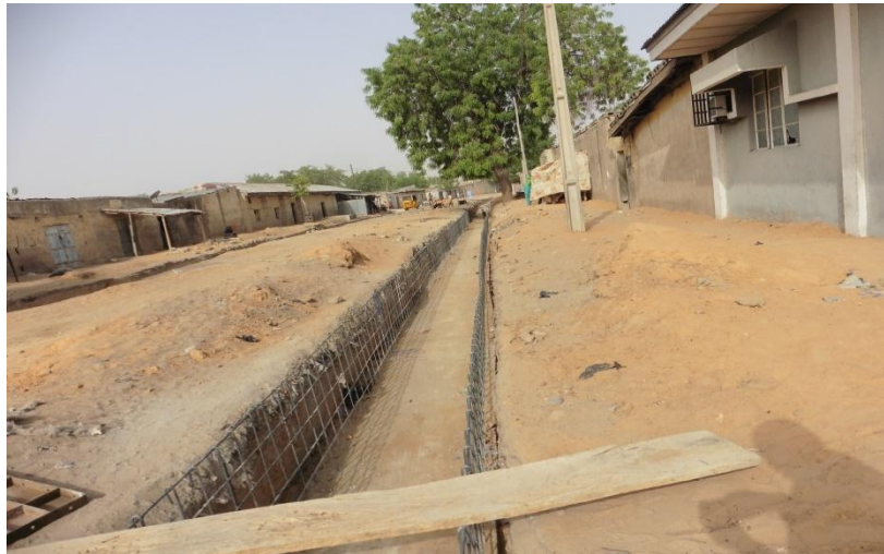
Figure 1:- Drainage under construction
