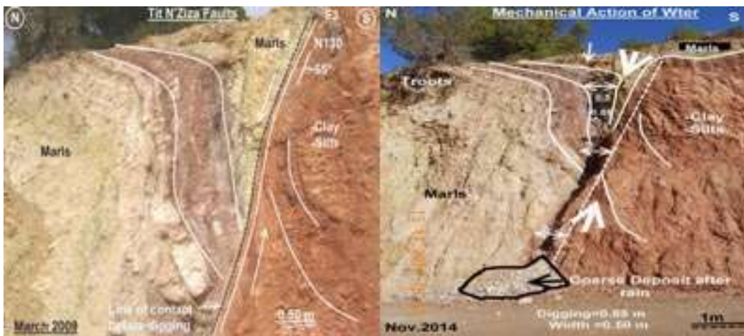
Fig 7:- Rainfall impact on weak structures in the slope
