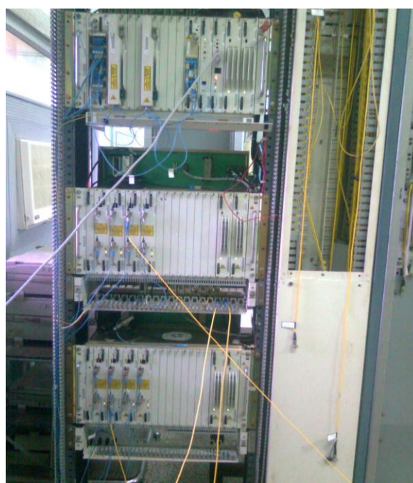
Figure 4: DWDM system components.
