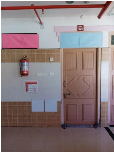
Figure no.1d; Room was completely closed
