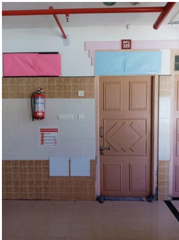
Figure no.1d; Room was completely closed
