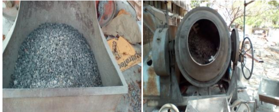
Fig.6 Mixing of materials.
